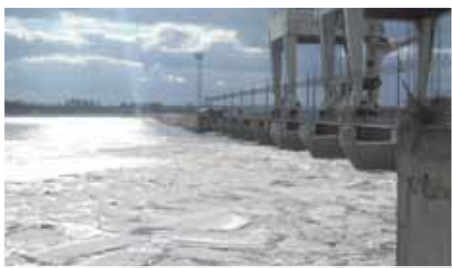
Plavinas HPP Upstream
